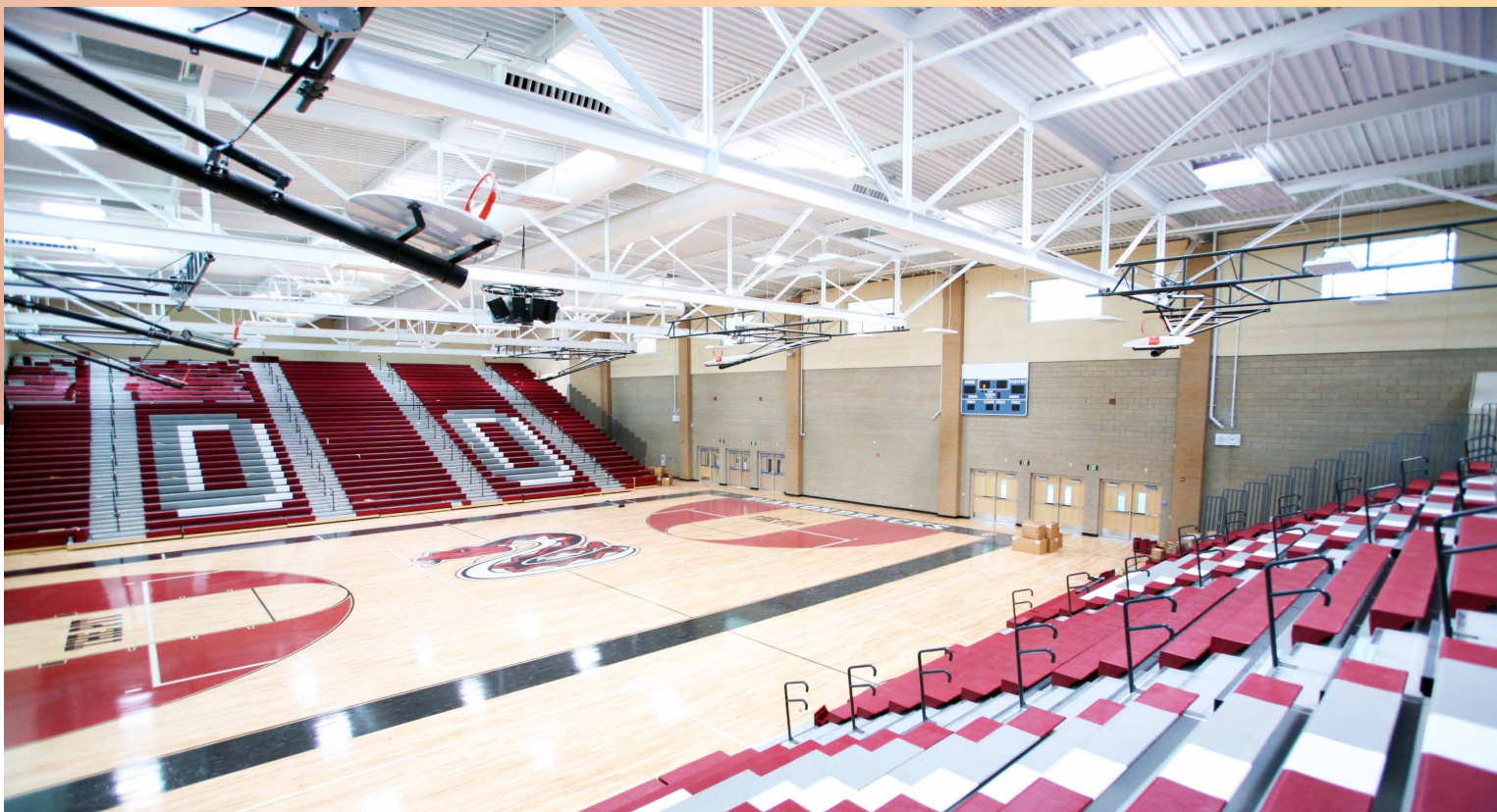
This High School Gymnasium in Las Vegas, NV is lit entirely by Ciralight SunTrackers. The electrical lighting is off!
