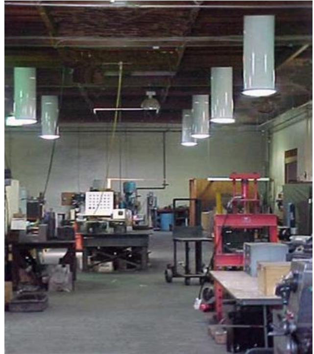
Suspended tubular skylights in this machine shop provide natural light for close-work visibility.
