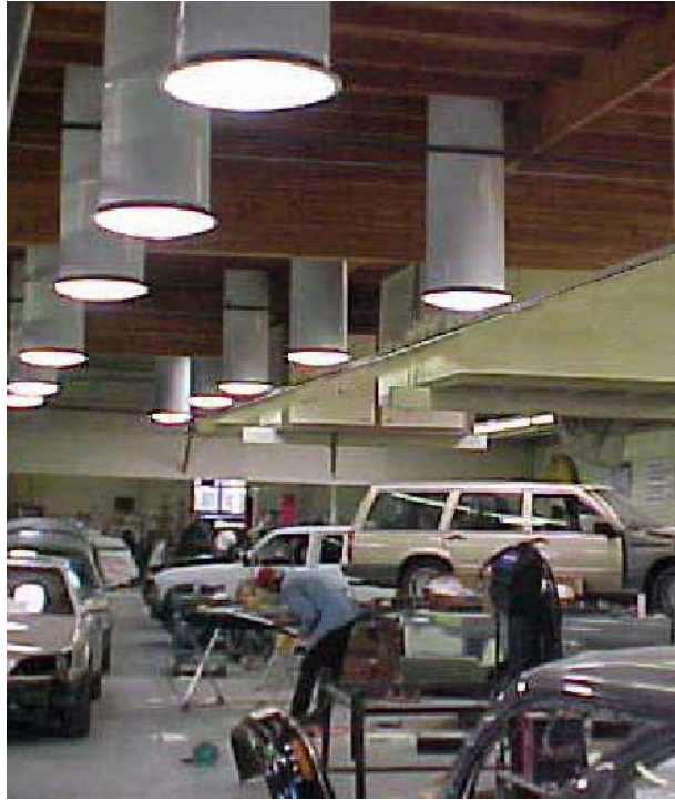
Suspended tubular skylights in this auto body shop render natural light that is perfect for matching paint.
