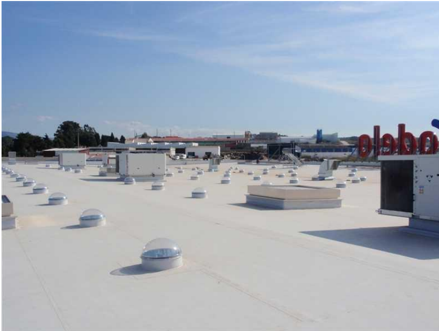
This installation is on a flat metal deck roof with insulation.
