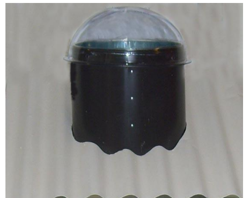
This installation is on a corrugated metal roof.
