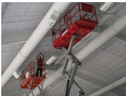
Installation of EverLast® 400w High Bays
