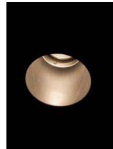
Figure 2.11. Closeup of recessed PAR30 downlight in Conference Room. www.kenricephoto.com
