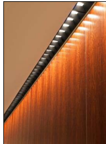
Figure 2.28. Closeup of wall grazing lighting (LED). www.kenricephoto.com
