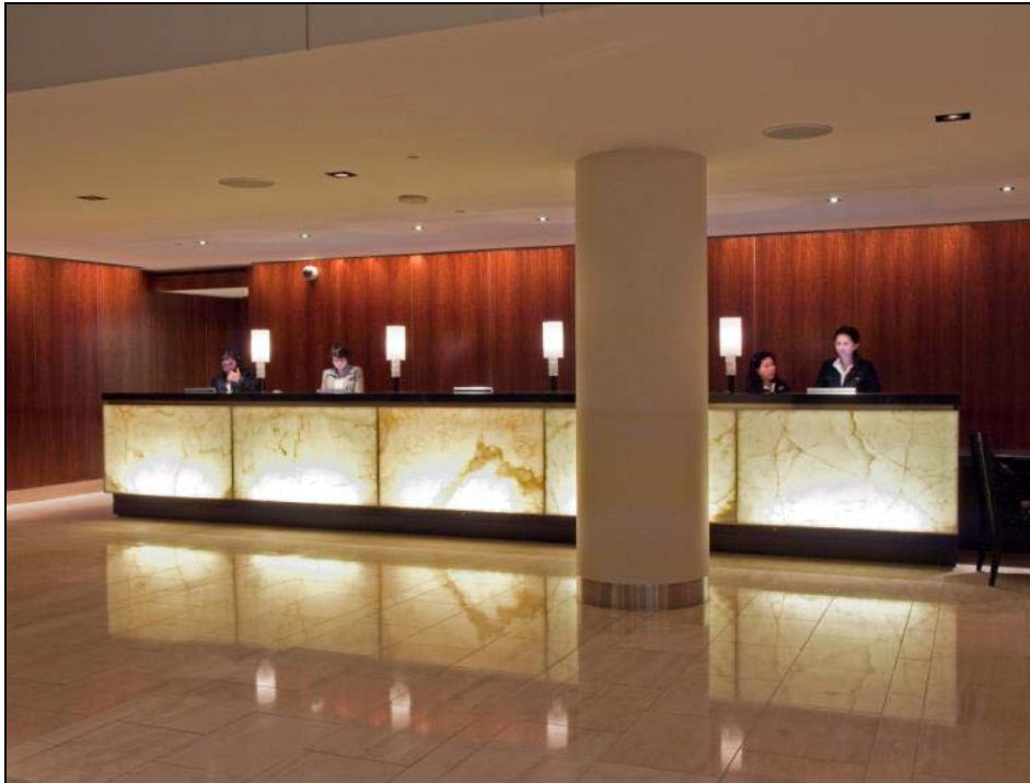
Figure 2.24. Registration Desk area with halogen accent and wall-grazing (onyx panels are backlighted with fluorescent lamps, and the pedestal lights use incandescent lamps). www.kenricephoto.com
