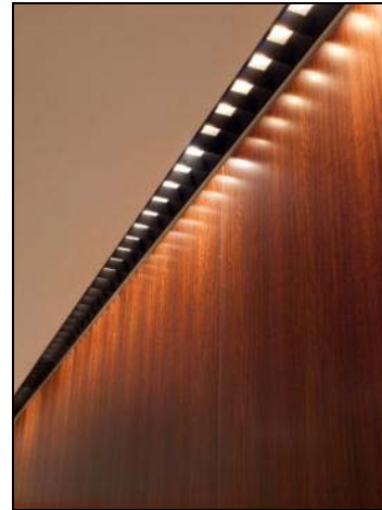
Figure 2.27. Closeup of wall grazing lighting (Halogen). www.kenricephoto.com
