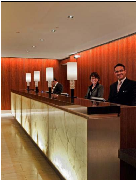
Figure 2.27. Registration Desk area counter showing overhead accent lights with LED replacement lamps. www.kenricephoto.com
