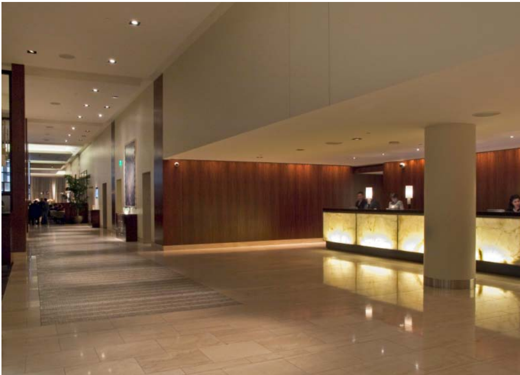
Figure 1.1. Photo of InterContinental Hotel Lobby with Original Halogen Lamping in Registration Desk Area. A complete relamping of halogen lamps was carried out to ensure optimum light output. www.kenricephoto.com
