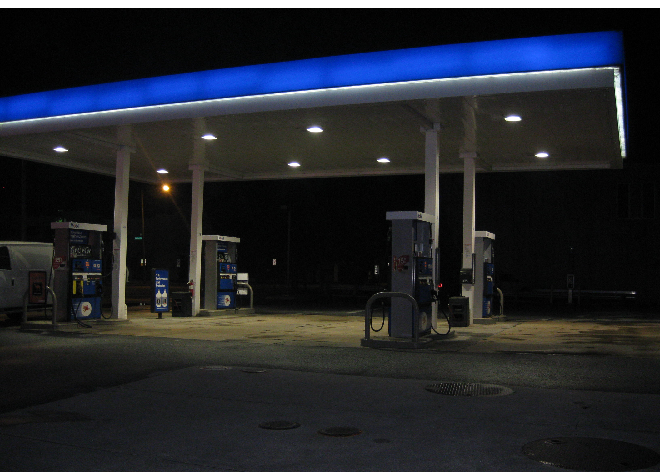
Before LED retrofit
