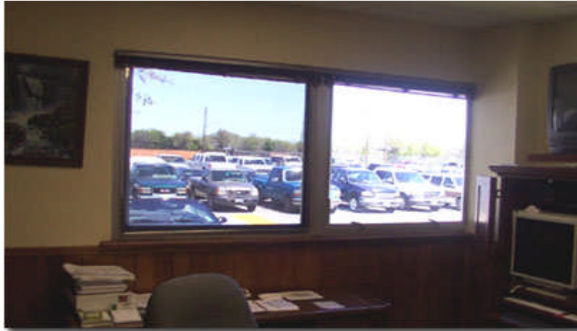
Left Side: Eco-Flector Panel Installed Right Side: No Eco-Flector
