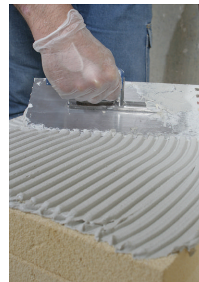
apply with notched trowel (entire surface)
