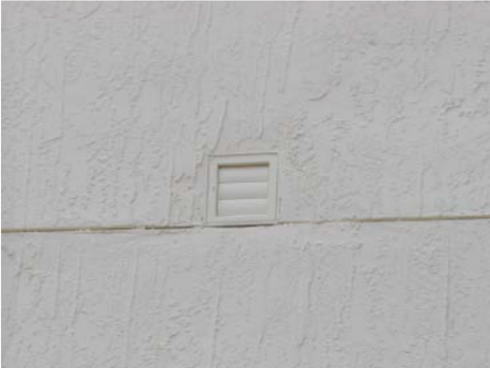
Photograph 34: Dryer Vent Opening
