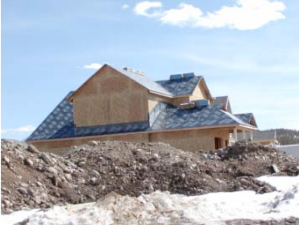
Photograph 72: Direct Applied Self Adhering Membrane
