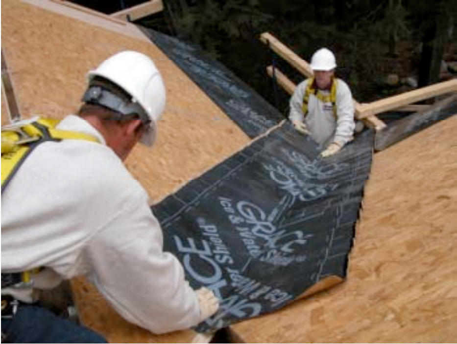
Photograph 71: Self Adhering Membrane
