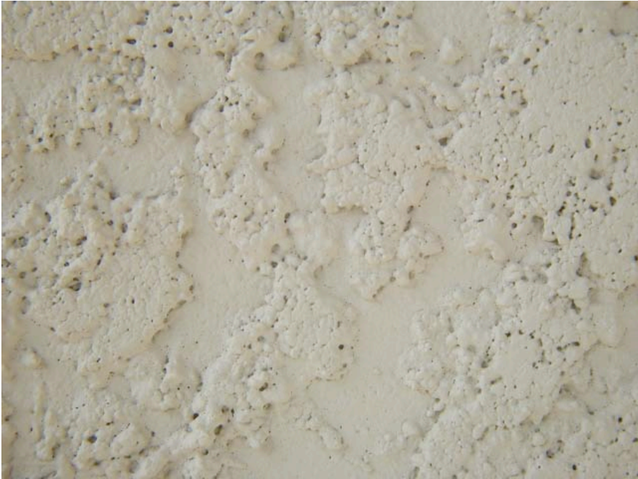
Photograph 67: Paint Coating – 3 Mil Thickness
