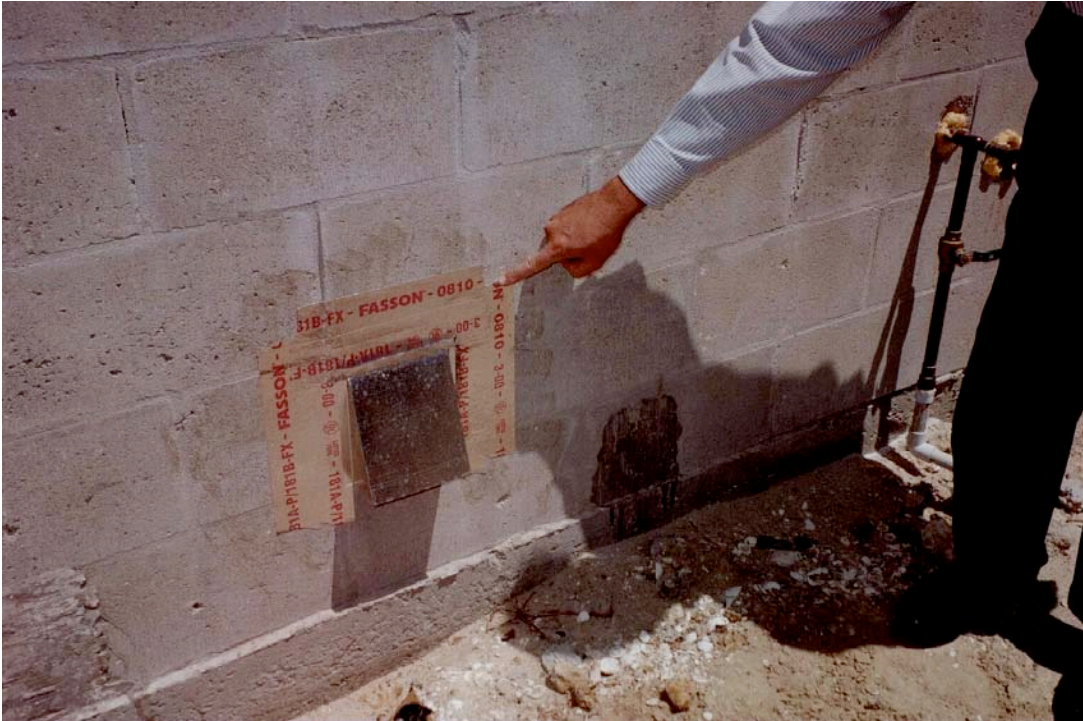
Photograph 36: Flashed Electrical Box
