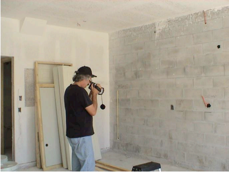
Photograph 44: Infrared Camera Leak Detection
