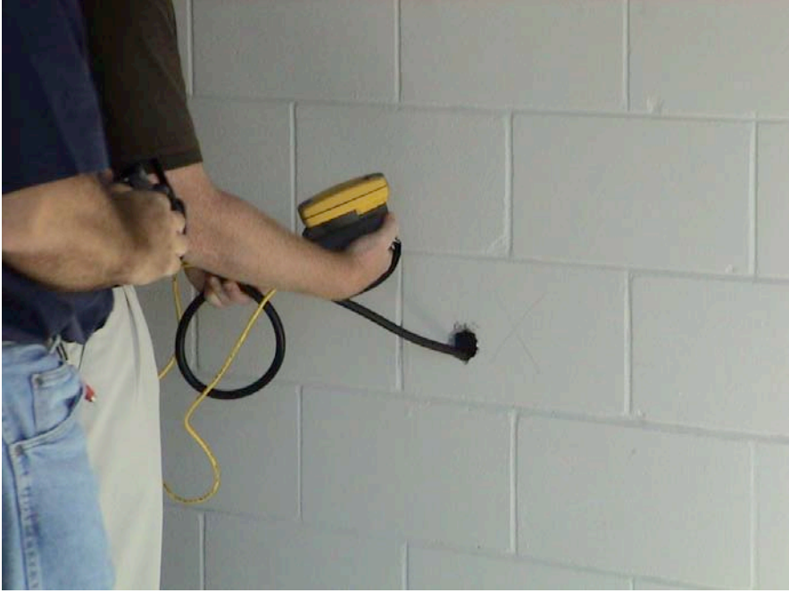
Photograph 45: Camera Probe Leak Detection
