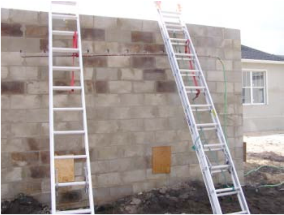
Photograph 54: Spray Rack Without Induced Pressure Difference
