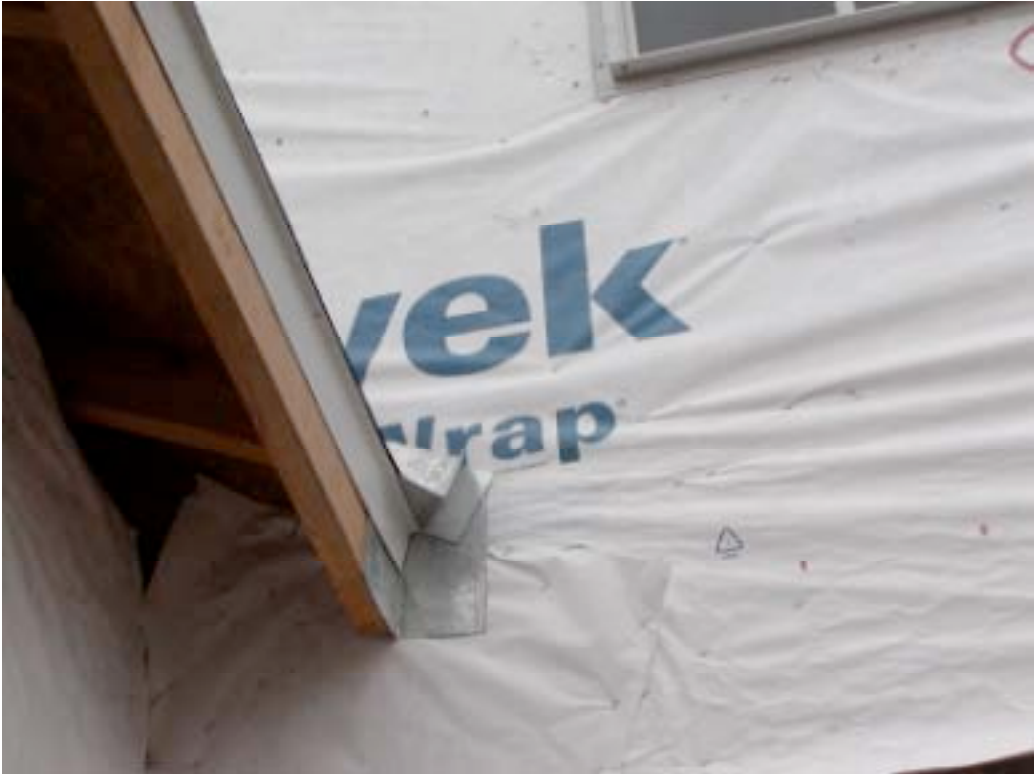
Photograph 38: Recommended KickOut Flashing Detail
