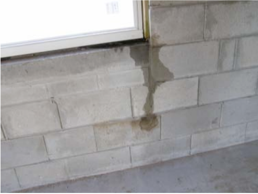
Photograph 24: Window Corner Leakage
