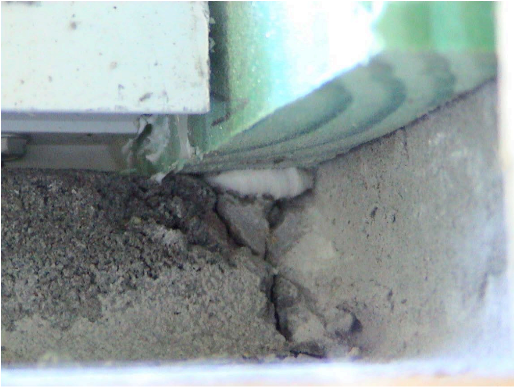
Photograph 26: Mulled Window Unit Leakage Paths
