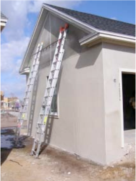
Photograph 59: Water Testing – Control Joints
