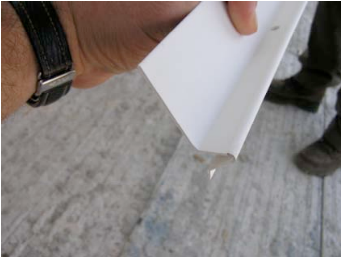
Photograph 18: Flashing/Control Joint - Weep Screed Flashing
