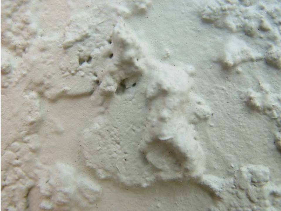
Photograph 68: Paint Coating – 10 Mil Thickness
