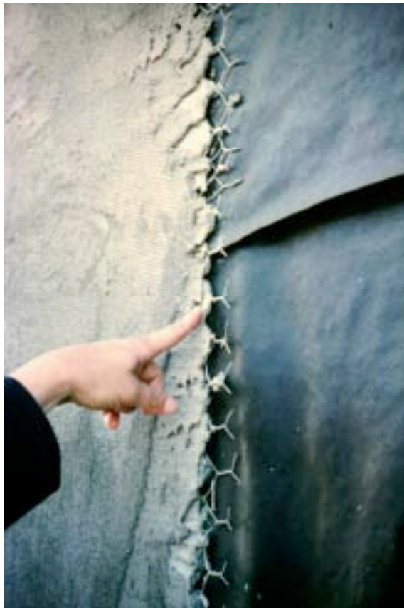
Photograph 3: Stucco Rendering Bonding to Building Paper
