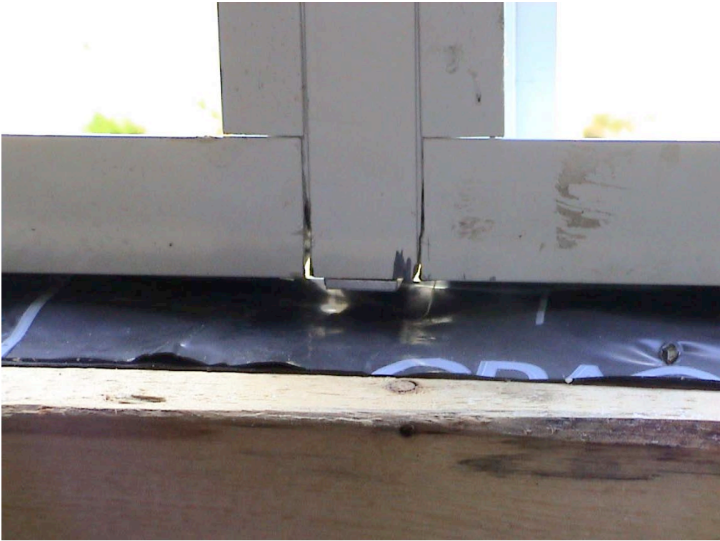
Photograph 26: Mulled Window Unit Leakage Paths
