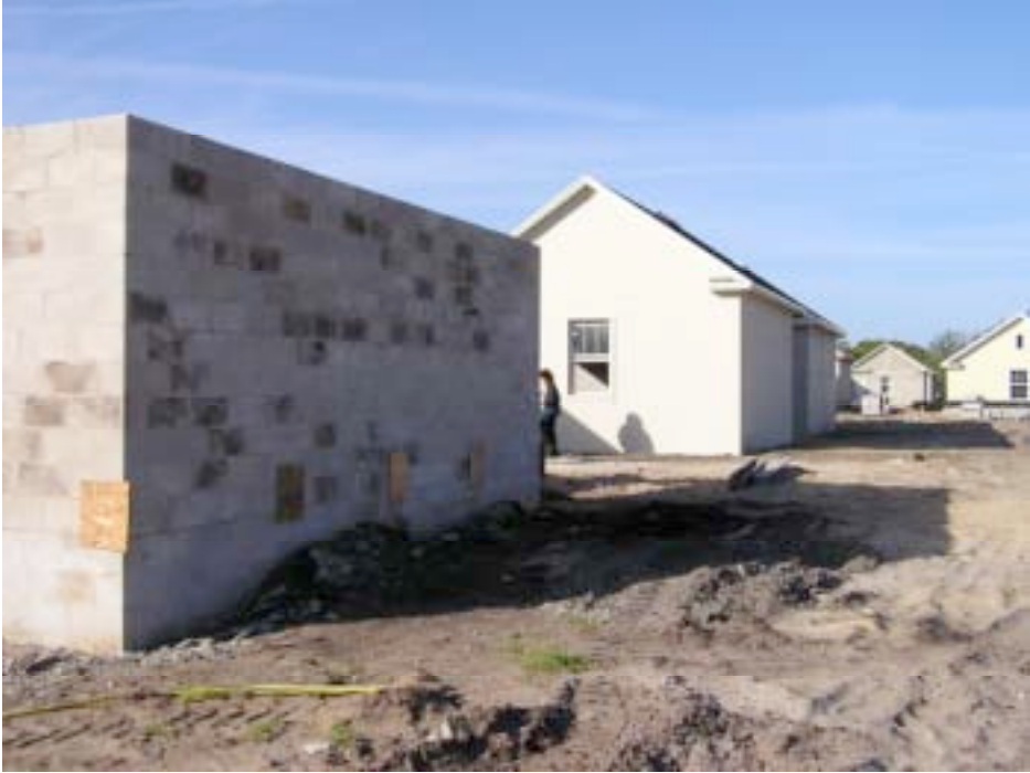
Photograph 51: Garages Used As Test Walls – Varying Configurations
