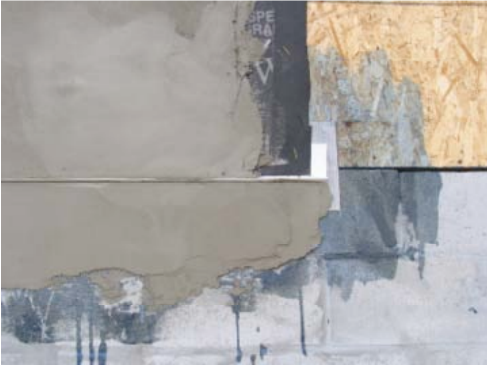
Photograph 22: Stucco Rendering Applied At Draining Control Joint
