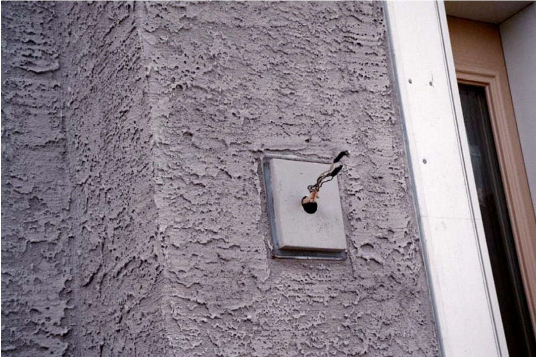
Photograph 36: Flashed Electrical Box
