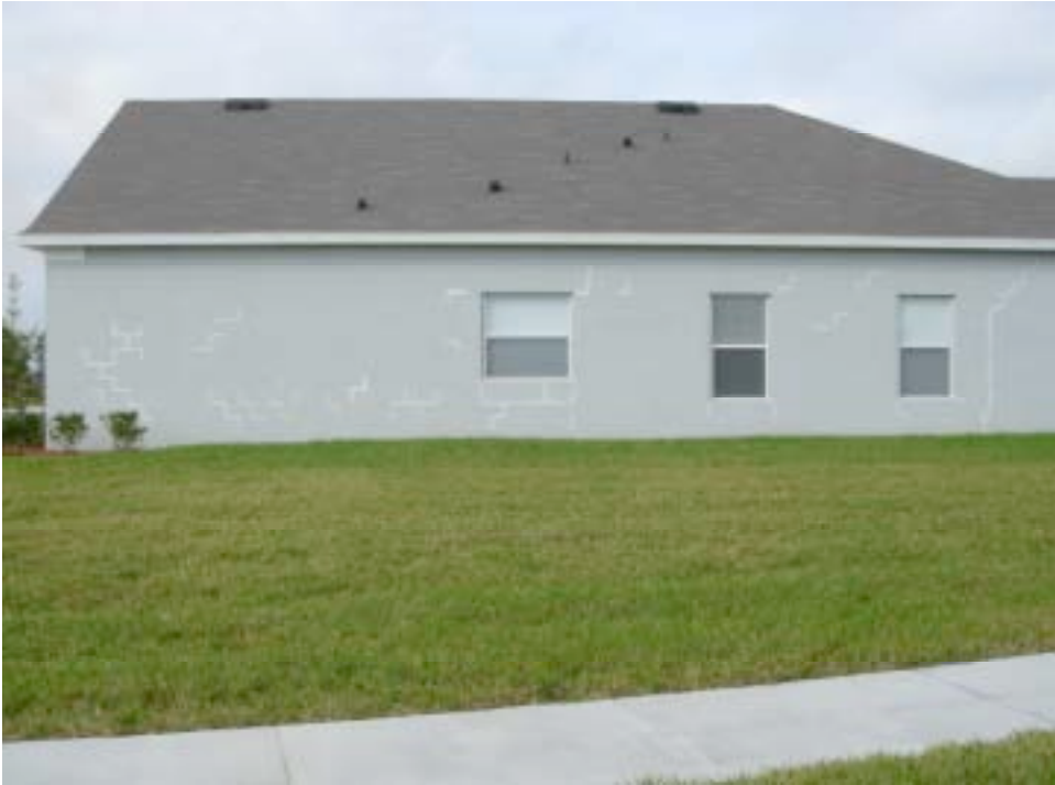
Photograph 70: Fiber Reinforced Stucco Rendering to Control Cracking
