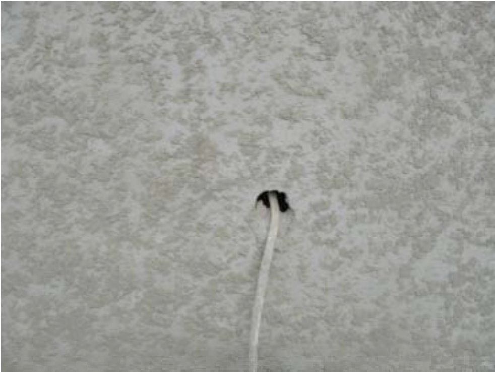
Photograph 32: Typical Maintenance Intensive Service Opening
