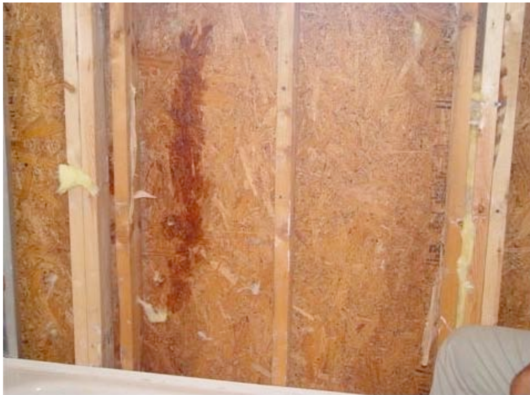
Photograph 2: Rainwater Entry into Second Floor Frame Assembly
