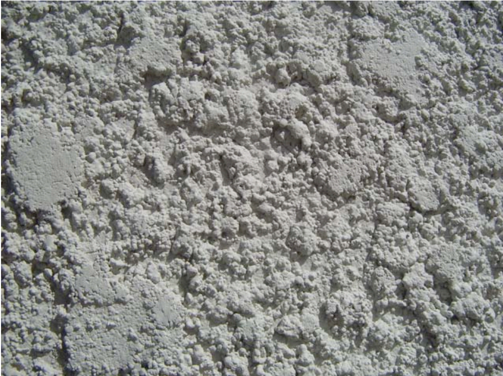
Photograph 66: Paint Coating Over Rough Surface
