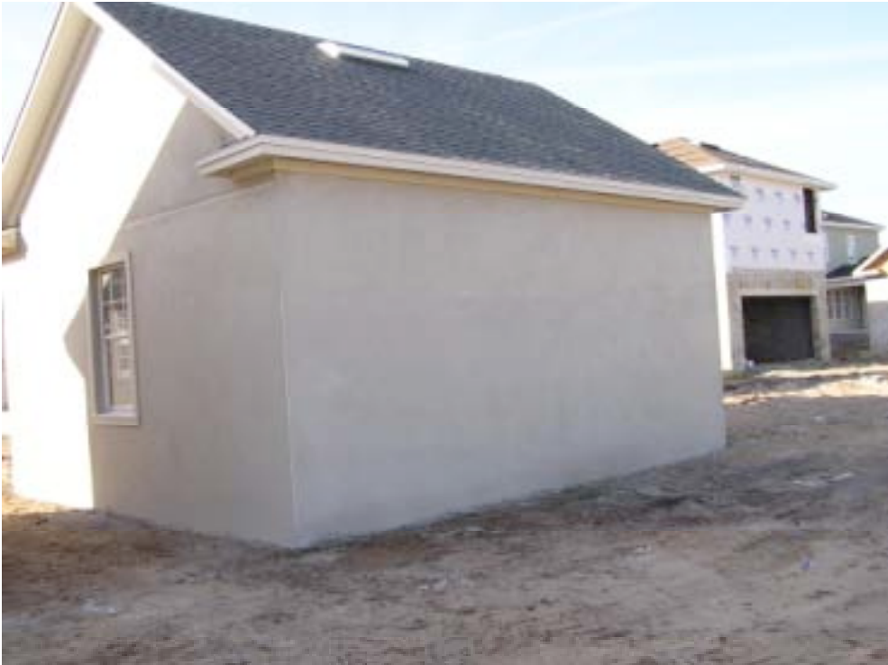
Photograph 53: Painted Stucco Rendering Test Wall
