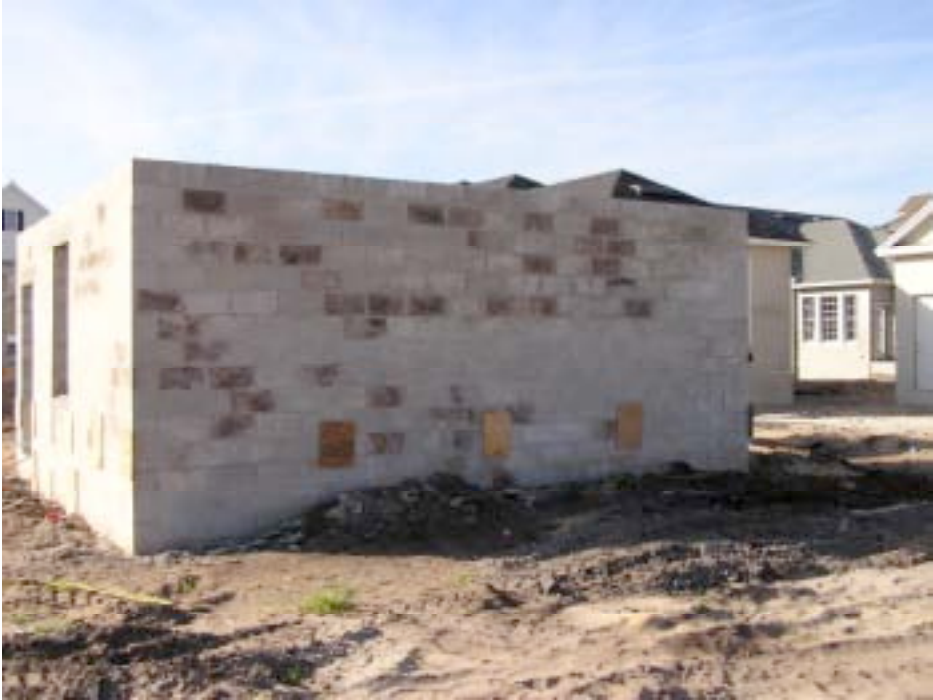
Photograph 50: Test Wall Establishing Baselines
