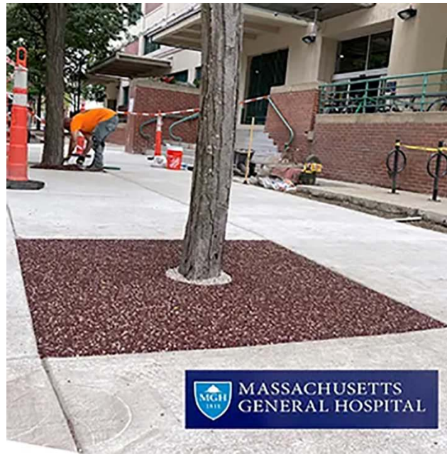
ELIMINATE TRIPPING HAZARDS.
