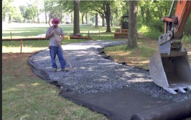
PLACE GEOTECH FABRIC AND STONE BASE
