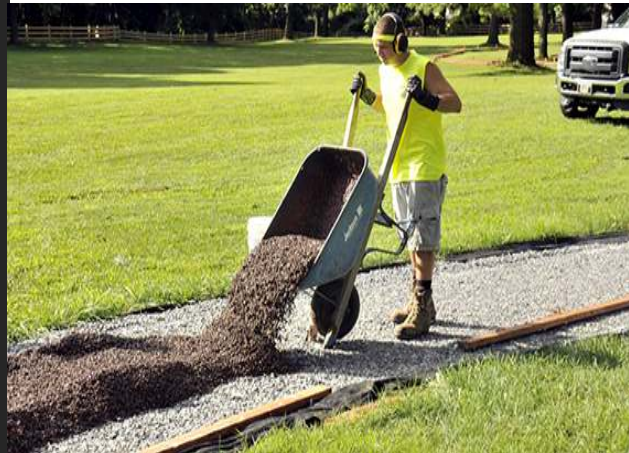
TRANSFER MIX TO POINT OF INSTALLATION
